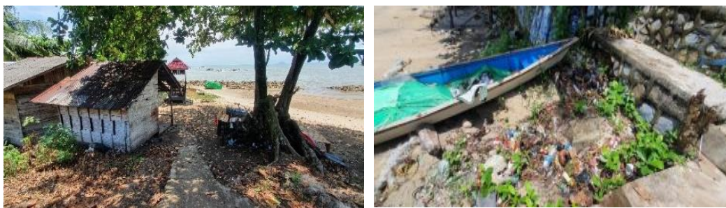
Figure 3. Unsuitable Residential Buildings and Waste Conditions Source: Field Survey Results (2022)
